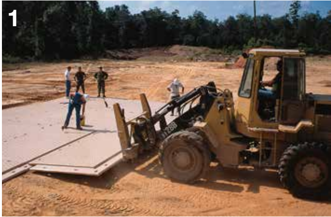
Mats are installed with standard site equipment.
