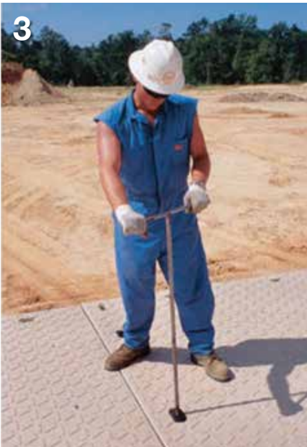
Pin fasteners lock mats into place to prevent separation.
